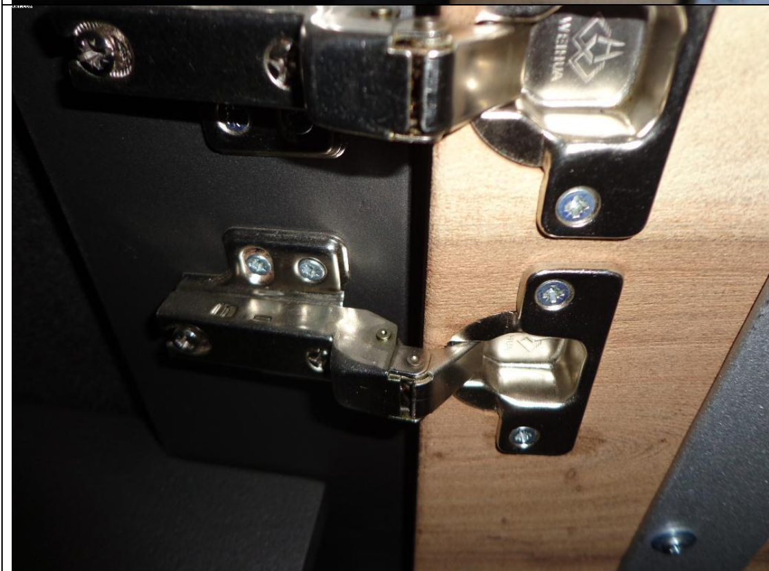
Adjustable soft closing hinges.
